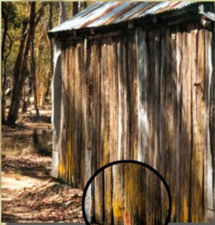
SLAB HUT: WOOD WALLS AND SUPPORTS
